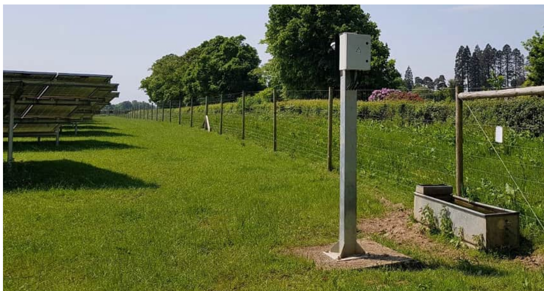
Plate 6. Typical mesh and wooden post perimeter fencing
