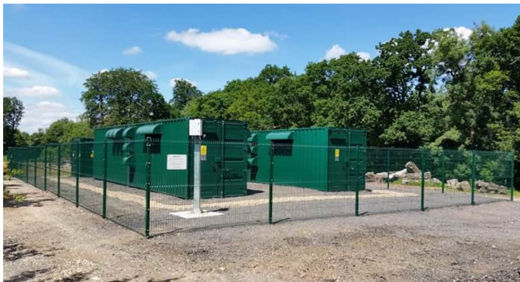
Plate 4. Typical pair of central inverters
